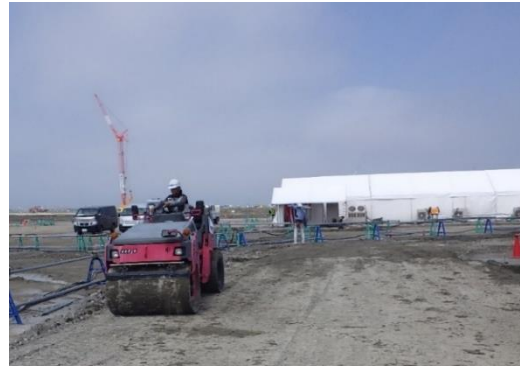
Ground improvement work in progress
