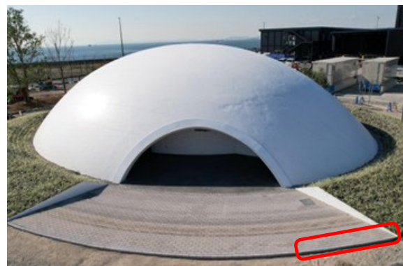
Entrance area of the Sustaina-dome where the pavers were installed
